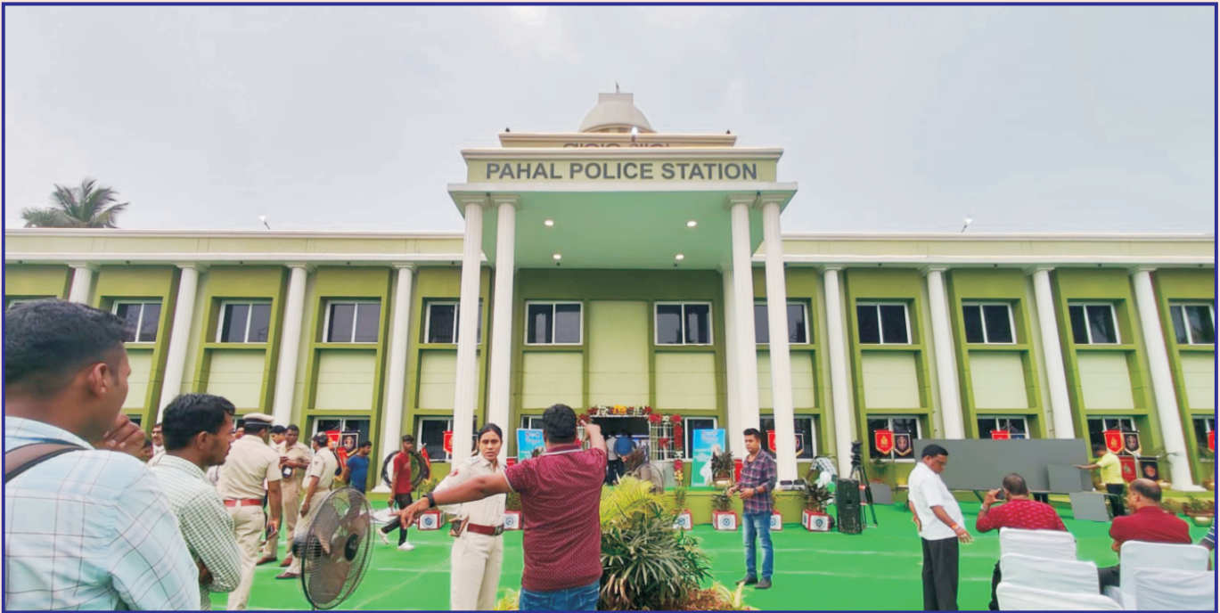
Pahal Police Station
