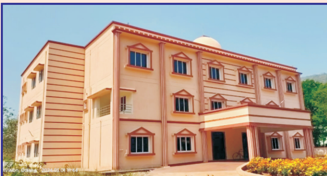
Admin Building PTS Nayagarh
