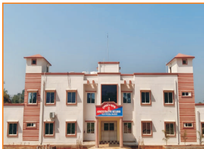
Administrative Building 3 rd SS Bn, Gajapati
