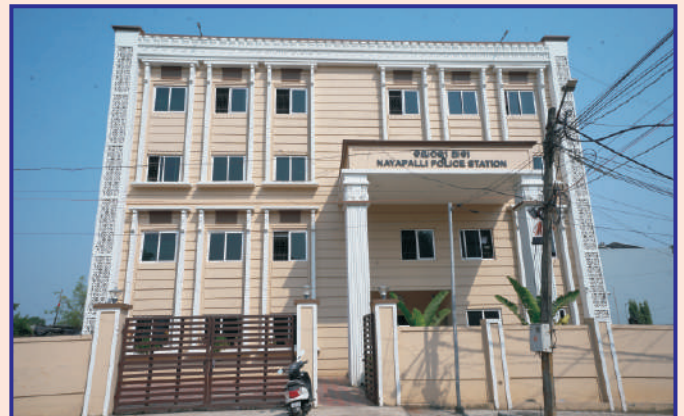
Nayapalli Police Station
