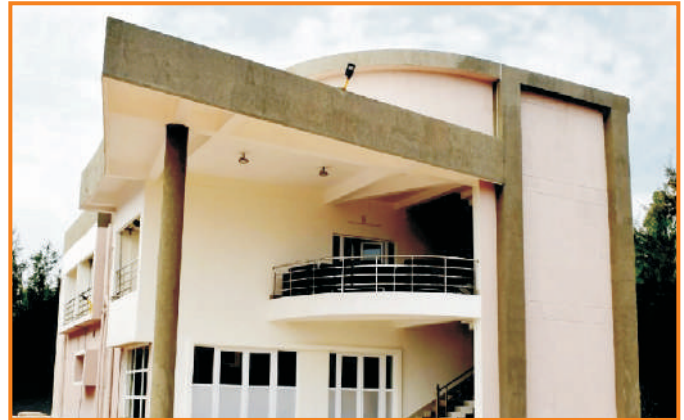
Kitchen cum Dining Hall OSWALI, Puri
